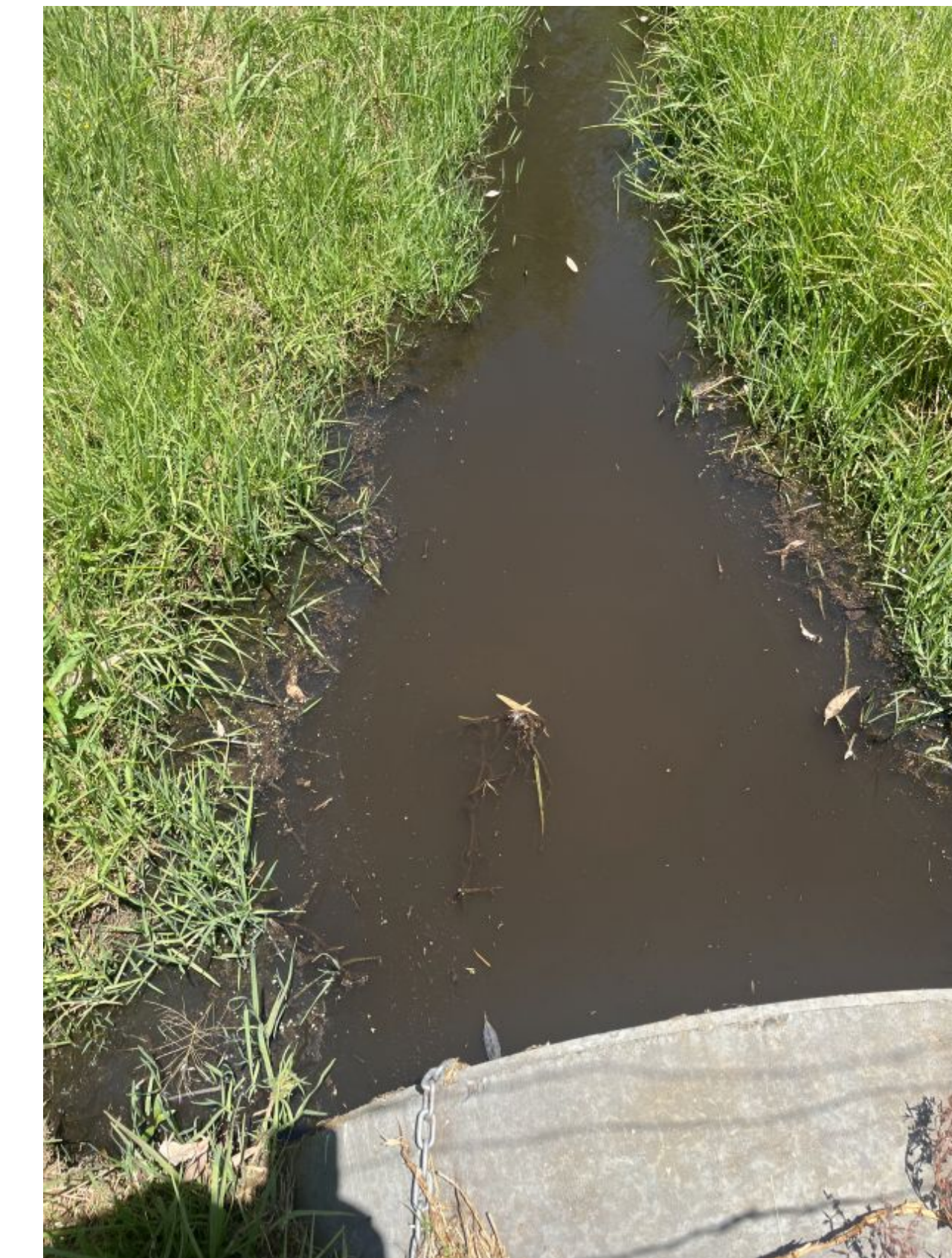
Water in culvert January 2026
