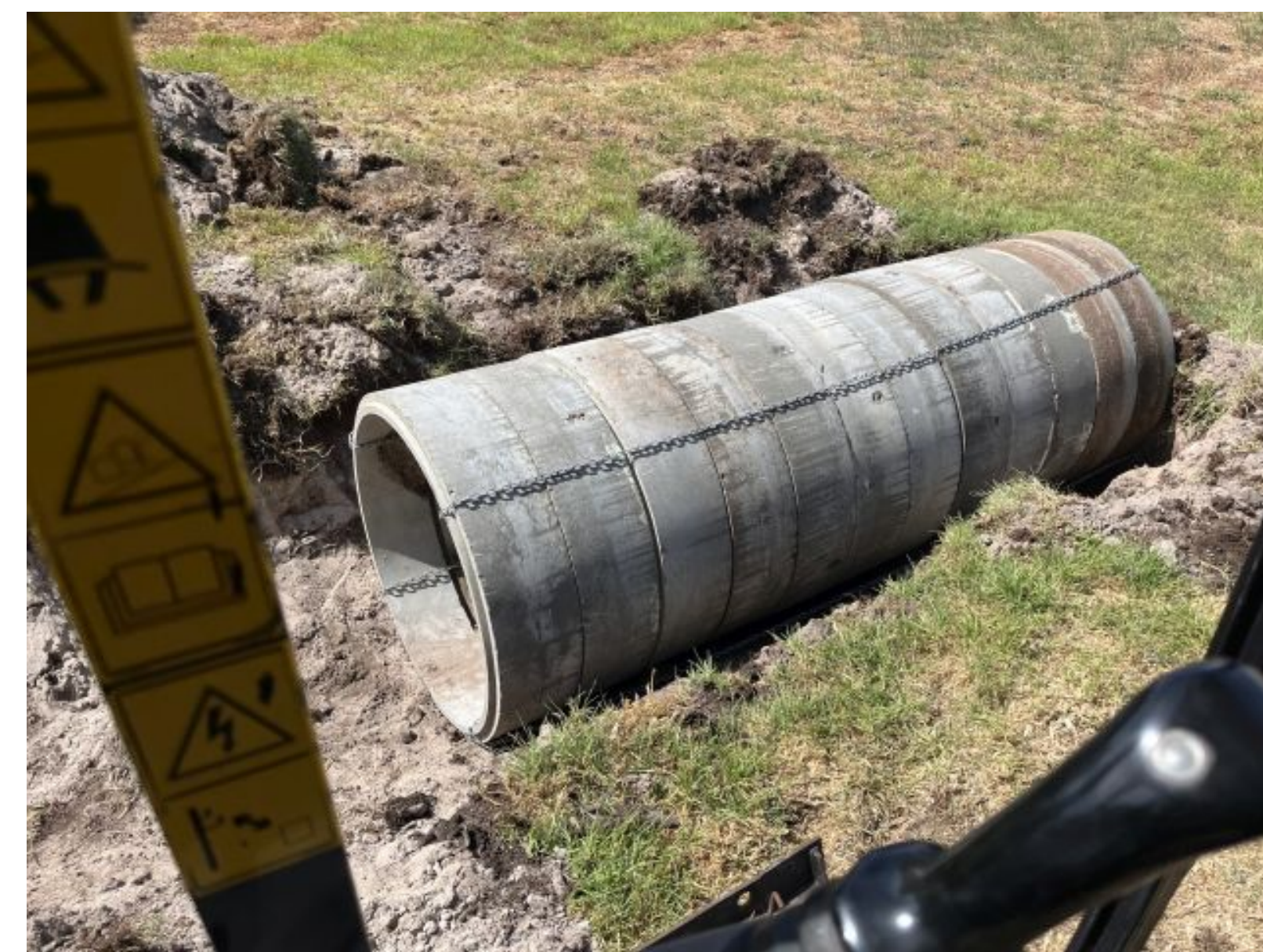
1.2m culvert installation January 2024
